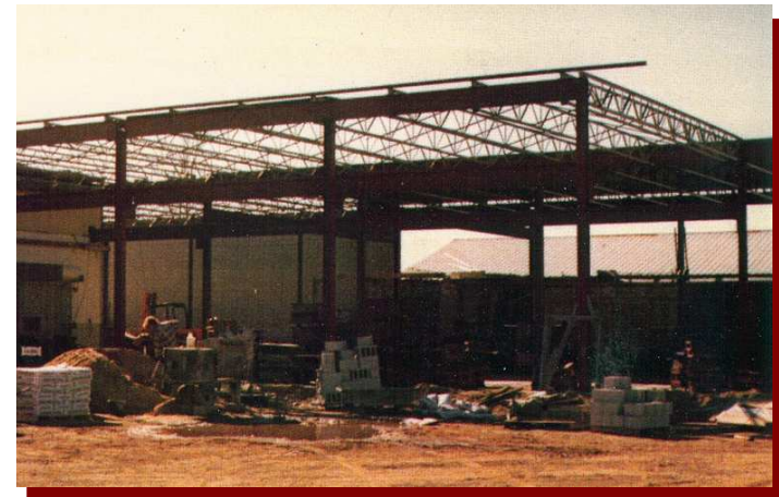
View of construction of the addition in-between two existing buildings
