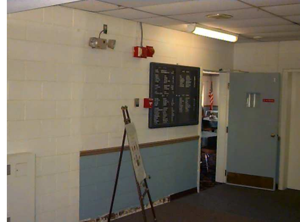
View looking at the existing Main entrance Dining Room before renovation.
