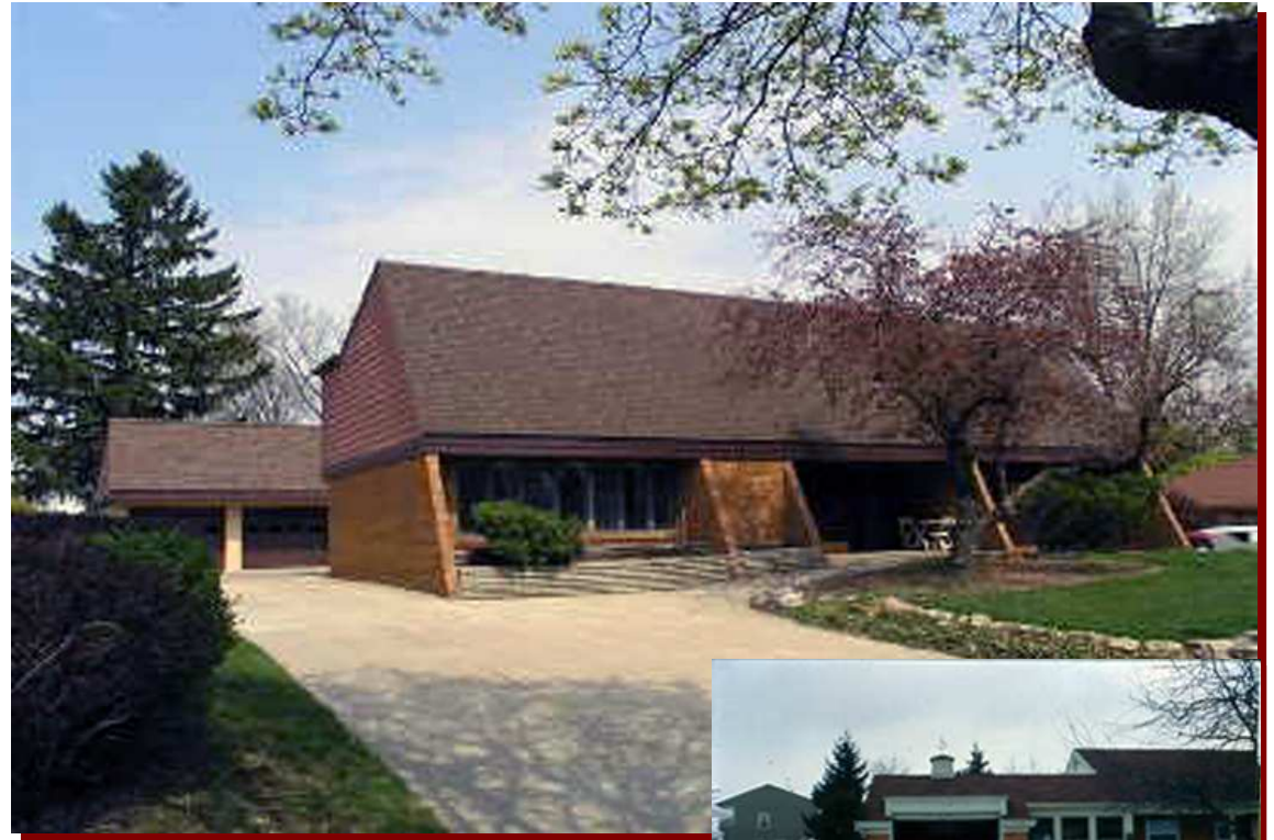
Photo of Addition after renovation
