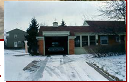
Photo of Addition area before renovation
